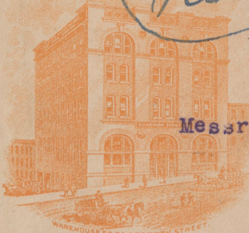
WAREHOUSE 52, 54 & 56 NINTH STREET.
